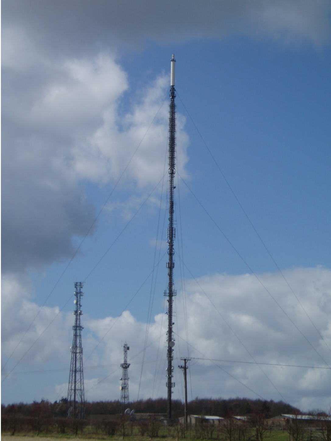
Photograph: 152m guyed mast near Beckley, Oxford 1
